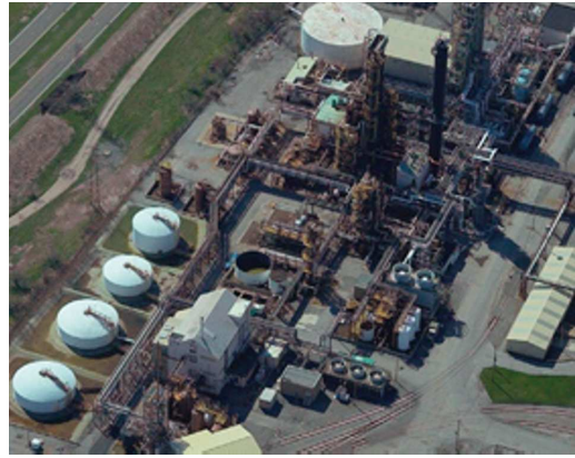
(b) Oil Refinery [13]
